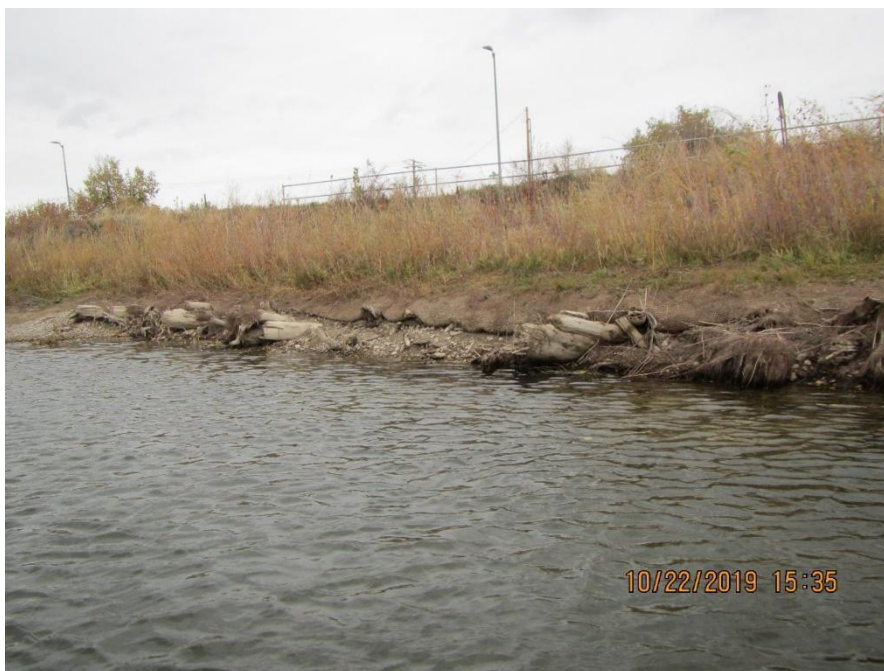
FIGURE A.5.6. Site 2 & 3 - Wyoming Blvd, at the middle of toe wood 3 in-stream, looking at downstream half of toe wood 3.
