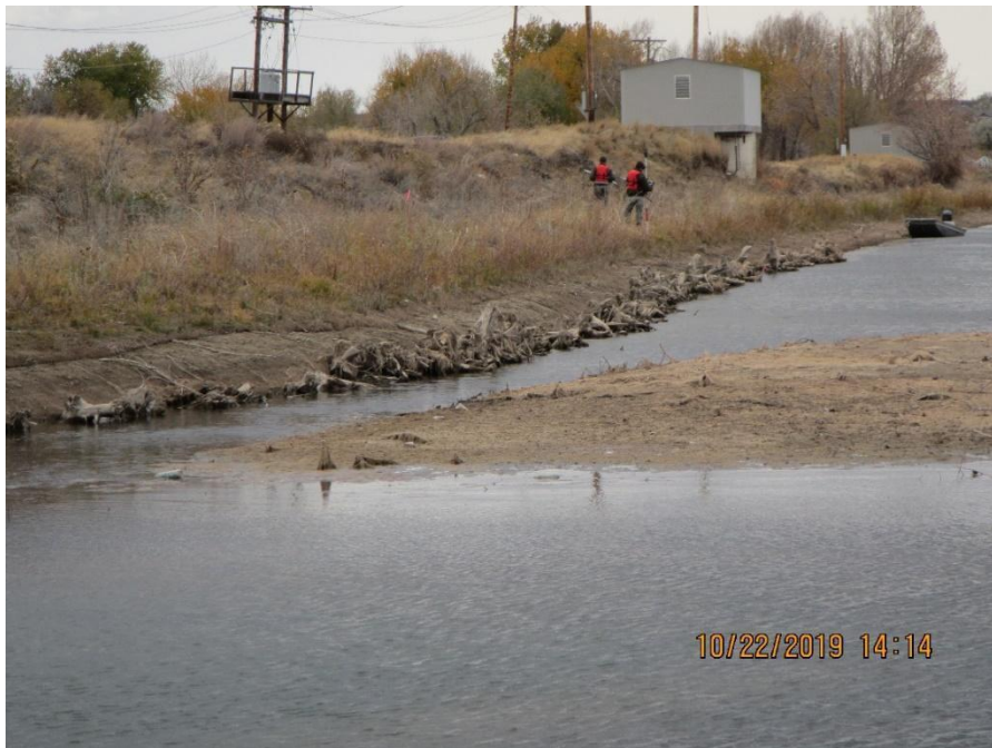
FIGURE A.5.10. Site 2 & 3 - Wyoming Blvd, standing in-stream, near upstream end of toe wood 5, looking downstream at lower half of toe wood 5.
