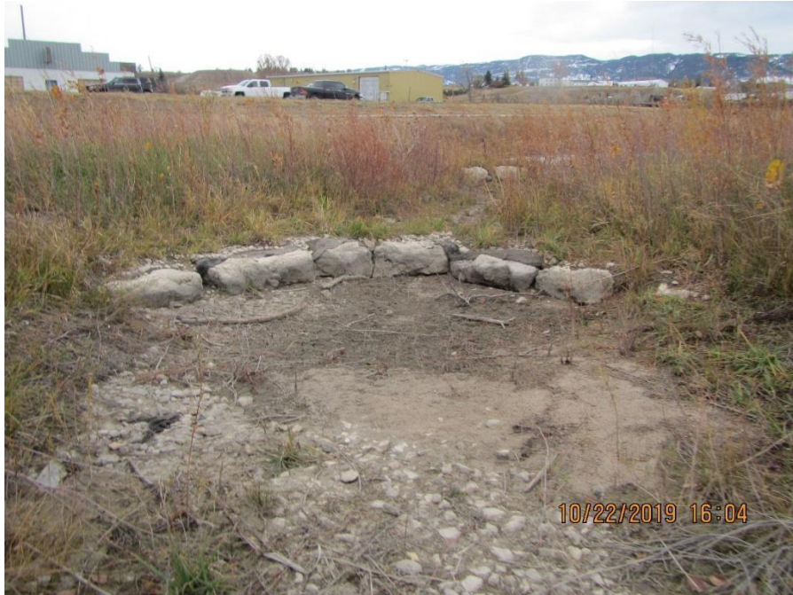
FIGURE A.5.21. Site 2 & 3 - Wyoming Blvd, at upstream set of wetland cross vanes, looking at cross vane 38.
