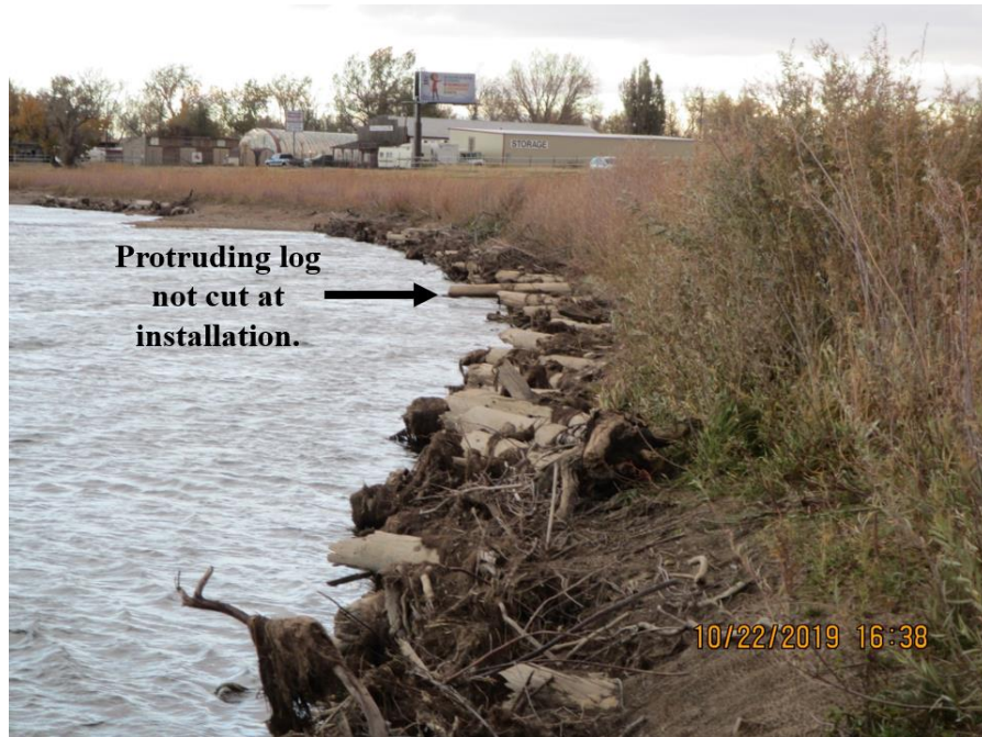
FIGURE A.5.1. Site 2 & 3 - Wyoming Blvd, standing near upstream end of toe wood 1, looking downstream.
