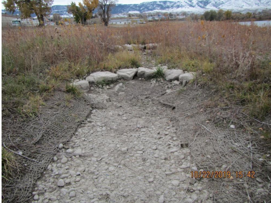
FIGURE A.5.25. Site 2 & 3 - Wyoming Blvd, at downstream set of wetland cross vanes, looking up at cross vane 41.
